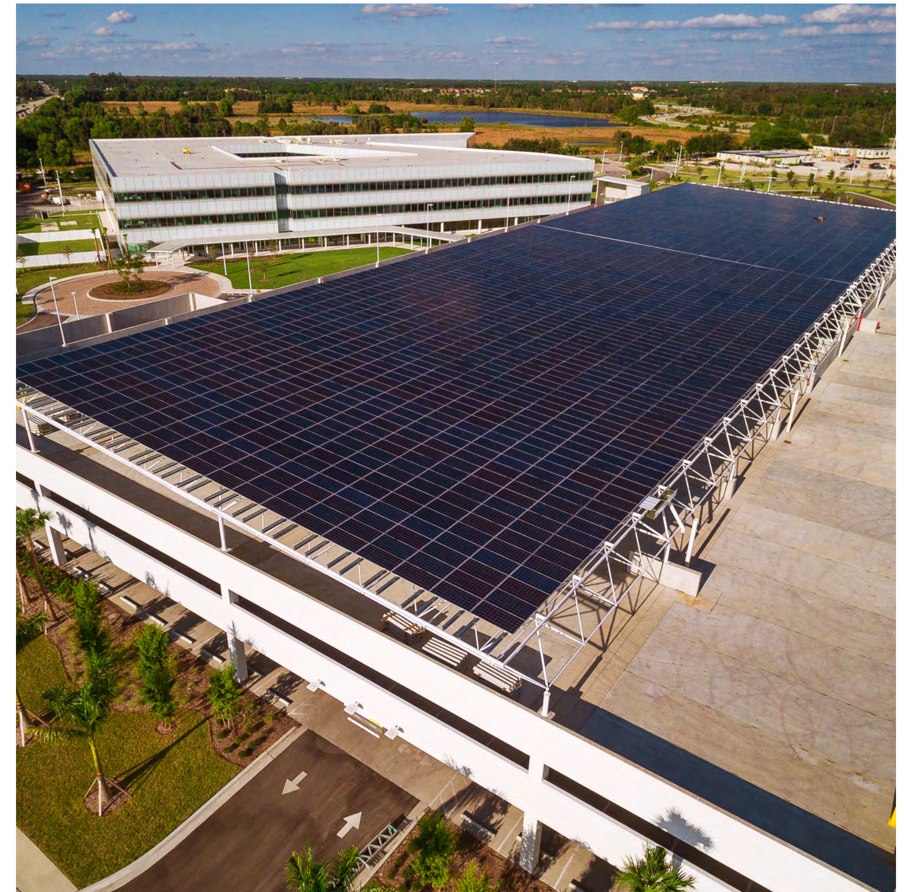
Solar array at Hertz HQ in Estero, FL.
